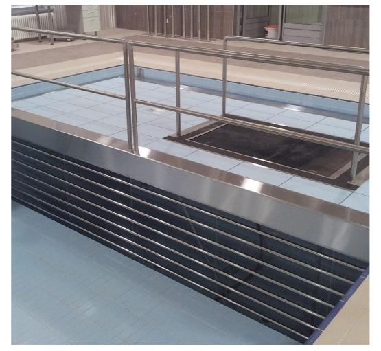
The suspended adjustable floor is used mainly in smaller therapy pools. The water depth can be adjusted to the patients needs. The EWAC Medical design concept
