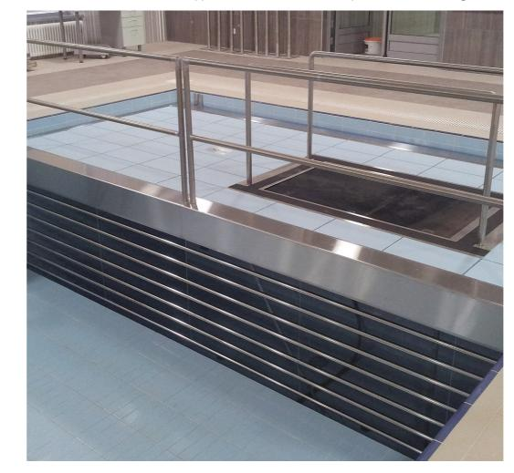
The suspended movable floor is used mainly in smaller therapy pools. The water depth can be adjusted to the patients needs. The EWAC Medical design concept
