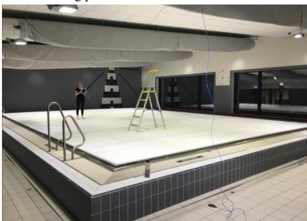
Figure 2 The swimming pool at Jøa with the moveable floor activated as a pool cover.
